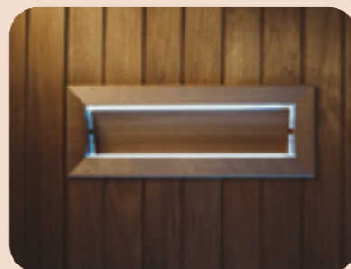
VENTILATION HATCHES For proper function of your sauna heater and for efficiency and longevity of your sauna, efficient ventilation is a must
